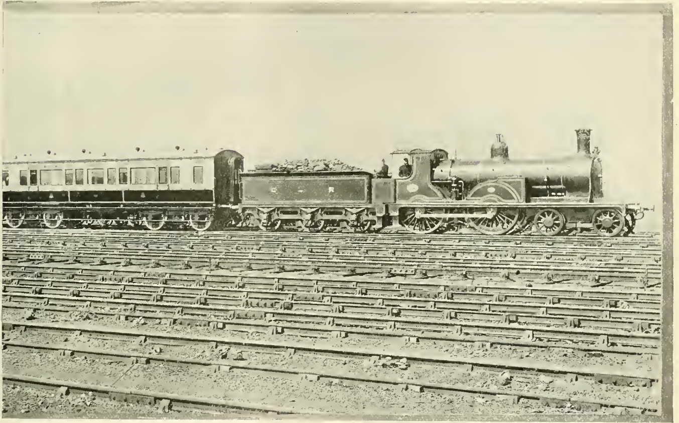
SHOWING FINE EXAMPLE OF TRACKS, BULL-HEAD RAILS.
